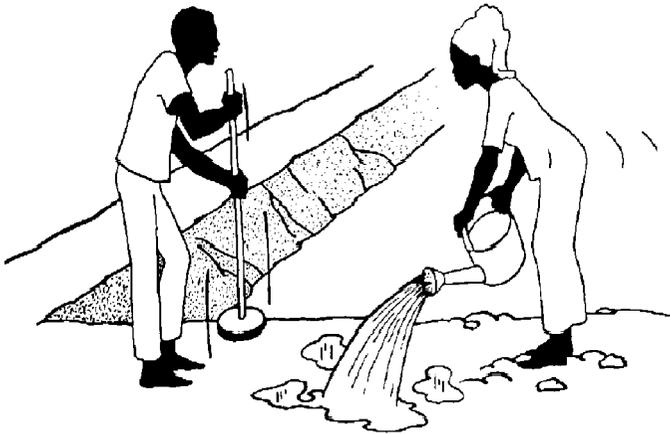
Figure 32: Compacting the dike (Viveen et al., 1985).
