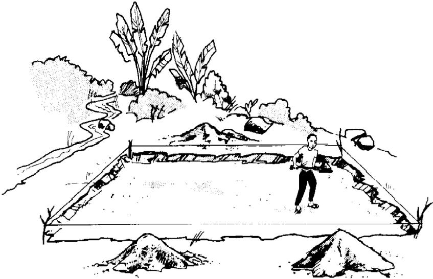
*Figure 29: Remove the top soil (Murnyak and Murnyak, 1990).*
